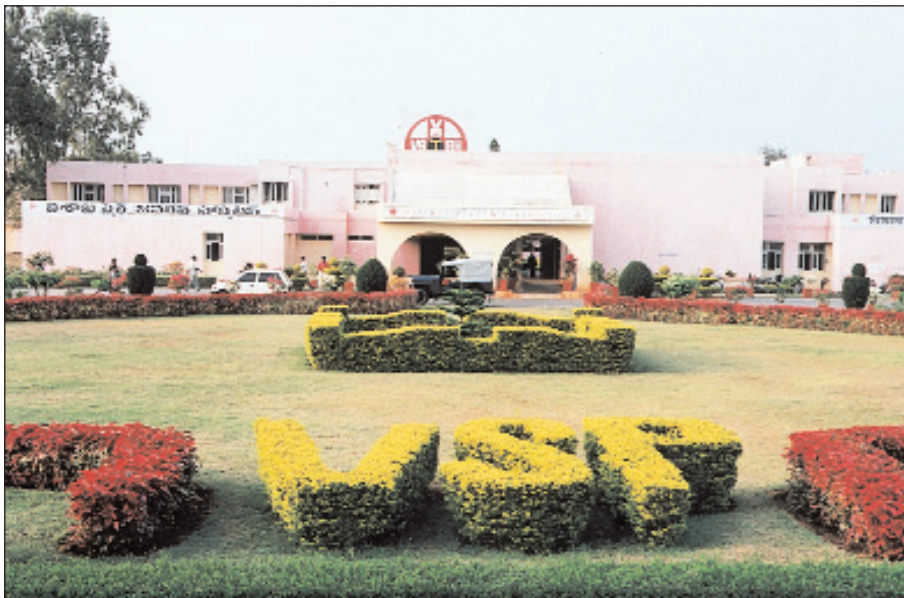
Visakha Steel General Hospital
